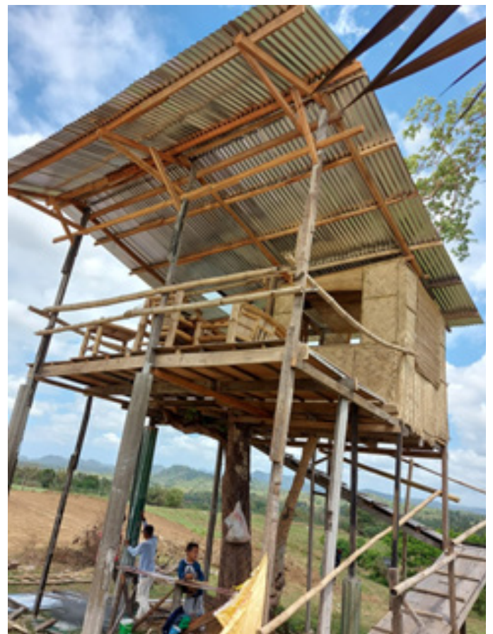
Construction progress to March 2021
